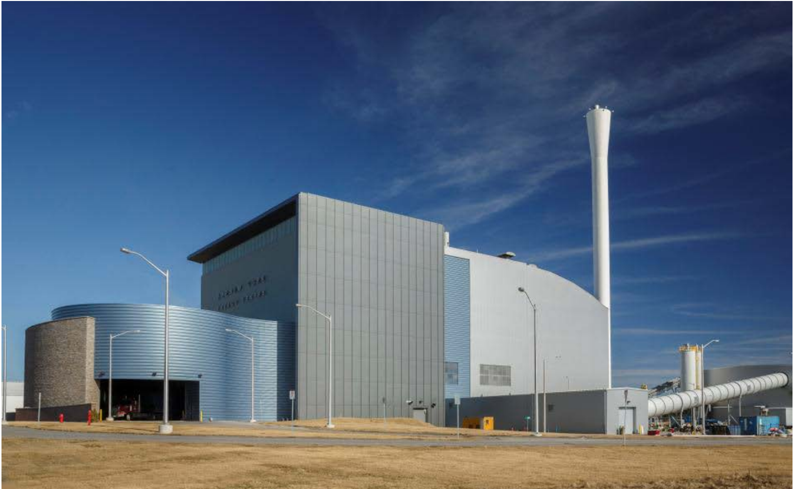
Durham York Energy Centre
